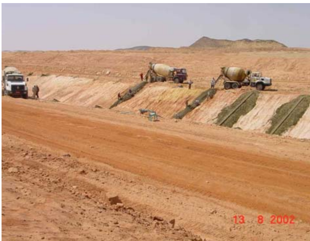
Constructing the canal
