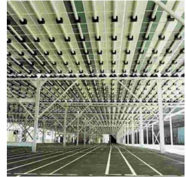
Shadowed usable area below flat mirror roof
