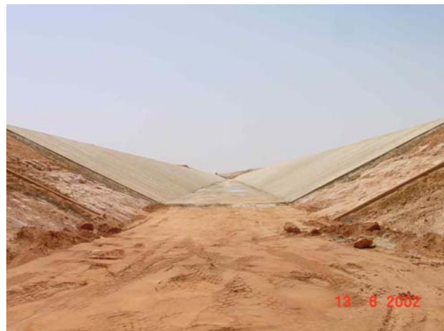
Lining the canal
